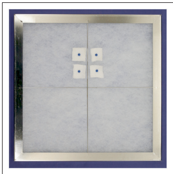
Figure 1. Gauze pieces pinned onto the exhaust air prefilter. With every new prefilter inserted into the air handling unit, four gauze pieces were pinned onto the prefilter to enable weekly collection of particle samples without having to change the exhaust air prefilter on a weekly basis.
